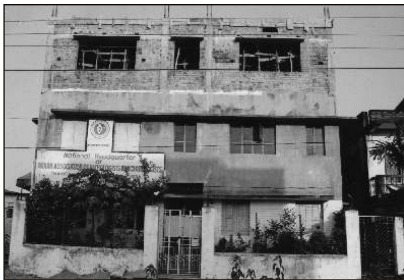
Recent photograph of the IAPM Headquarters building at Cuttack
